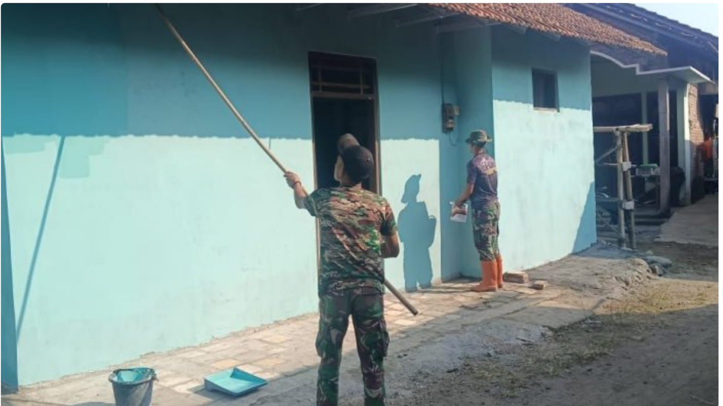
(Foto istimewa) Pengecatan RTLH TMMD 116 Kodim 0722/Kudus
